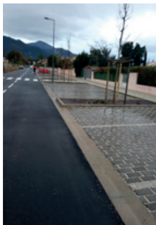
Parking Argelès sur Mer (source CD66)
